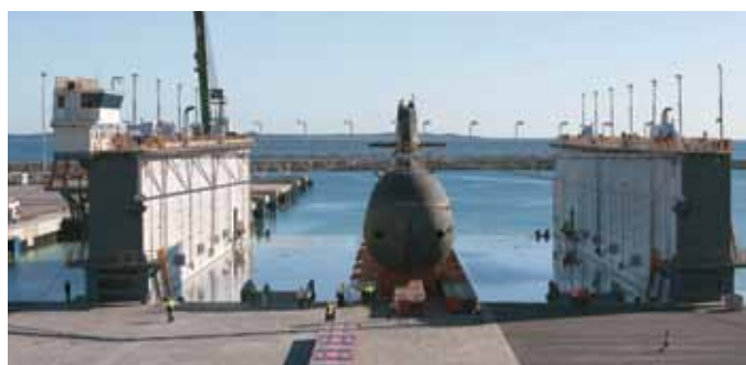
The first Collins Class submarine has been transported on the AMC floating dock.
