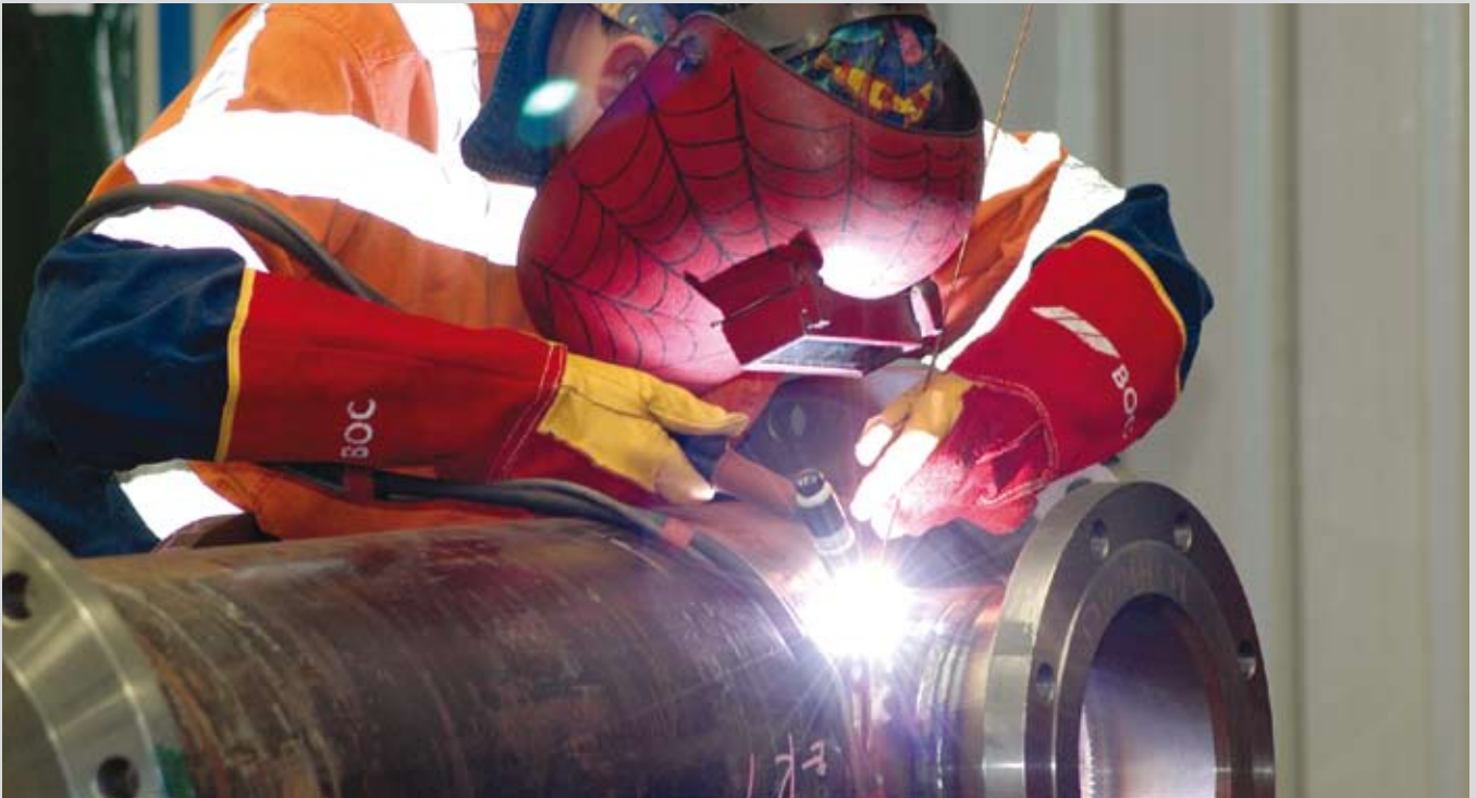
Link Weld Engineering will fabricate subsea tie-spools for the Pluto LNG Project.
